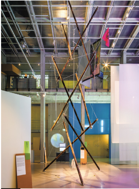
Fig. 3 The Beacon is held in place by the principle of tensegrity (a portmanteau for tensional integrity): The bamboo elements are compressed inside a network of tensioned cables. The removal or cutting of any piece of the structure leads to its collapse, making it hard to remove quickly. These structures have become useful architectural elements of protests around the world since their first use by Extinction Rebellion UK in 2019. The Beacon shown in the Nature of Hope exhibition space was assembled collectively with Extinction Rebellion Rotterdam and several activists from northern and central Europe.
